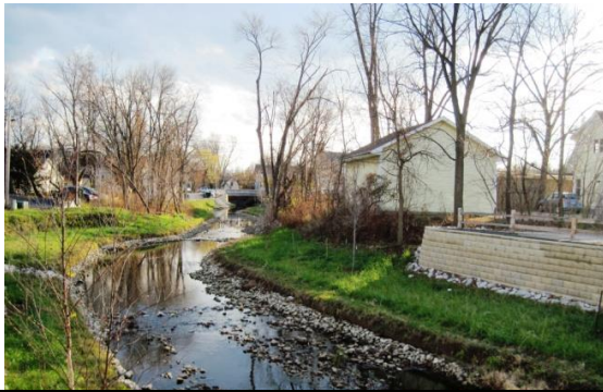
View of a portion of Pigeon Creek’s rock lined low flow channel and newly constructed retaining wall.
