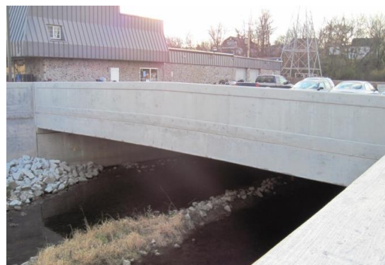
Photo of clear span bridge that replaced culverts
