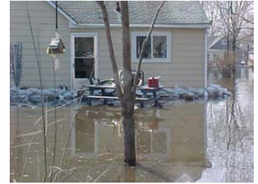
Dislocation of families from their homes is a common occurrence during flooding events. Dislocation costs are often times paid for by FEMA.
