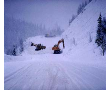
There were 253 snow and ice storm events in Wisconsin from January 1993 through June of 2000 causing two deaths, 47 injuries and reported property damages of over $770,000.
