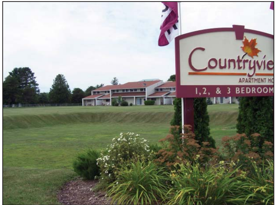
The Villa East detention basin alleviates flooding in the parking lot and buildings of the Countryview Apartment complex. Photo: Barbara Ellis, FEMA
