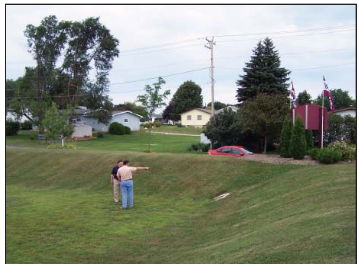
Alan Gerber, City Engineering Supervisor at the Department of Public Works of Monroe, Wisconsin, points out the direction of flow water takes when draining from the Villa East detention basin. Photo: Barbara Ellis, FEMA
