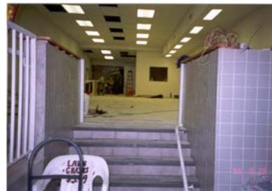
When flooding is imminent, a flood shield slides into a frame at the top of the steps, creating a solid, sealed floodwall. The street level vestibule was constructed with materials that would not sustain flood damage, like ceramic tile or brick. Floodwaters are allowed to enter in the area in order to equalize the water pressure avoiding structural damages.
