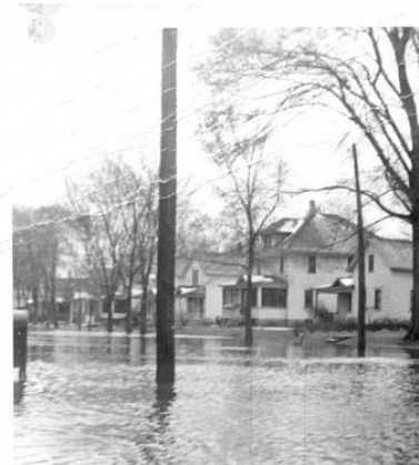
Upper left: Flooding on Forest St. and Madison in 1884.
