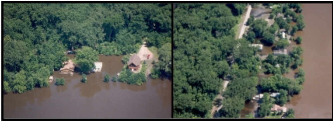
Shown above during the flood of 1993, many of these buildings were purchased and the lots returned to open space. The property owner of the two homes on the far left chose not to sell. The homes were flooded in 1997 and 2001.
