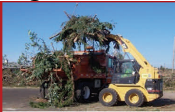
A. Debris Clearance
