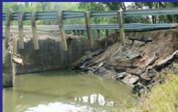
C. Roads & Bridges
